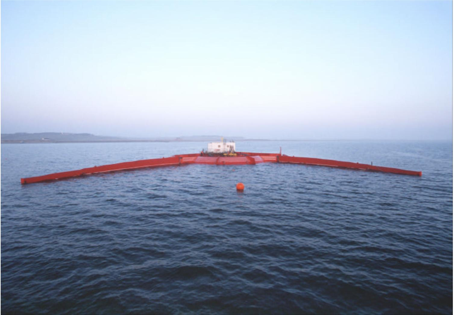
The Wave Dragon™ prototype (above) has been tested in real sea since March 2003. The white container is for test purposes.
